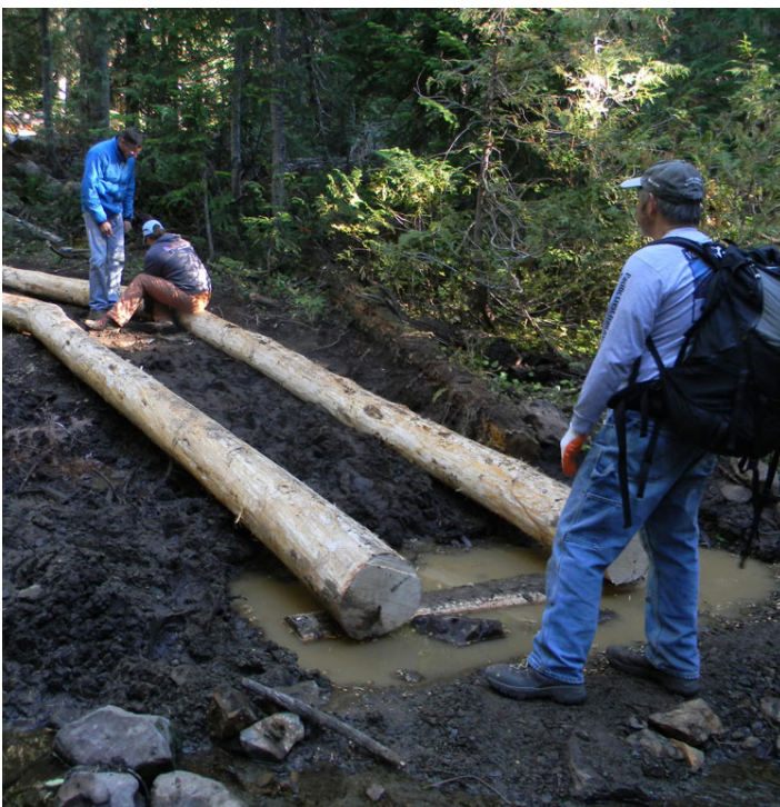
The Dark Meadow Trail on the Pacific Crest Trail is a popular loop that has suffered drainage issues. The Back Country Horsemen of Washington and the Pacific Crest Trail Association volunteers resolve the problem by constructing a turnpike to elevate the trail tread out of a wet area. Source: Deb Wesselius
